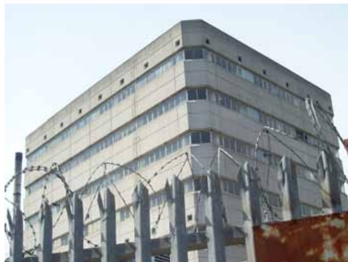
Rooftop potential for beehives at the derelict hospital Rory Walsh © RGS-IBG Discovering Britain
